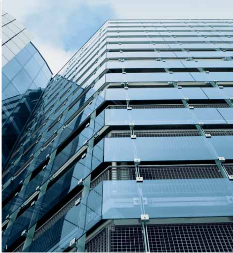
Hot-dip galvanized 1 press locked gratings Façade of a multi-storey car park Ulm/Germany
