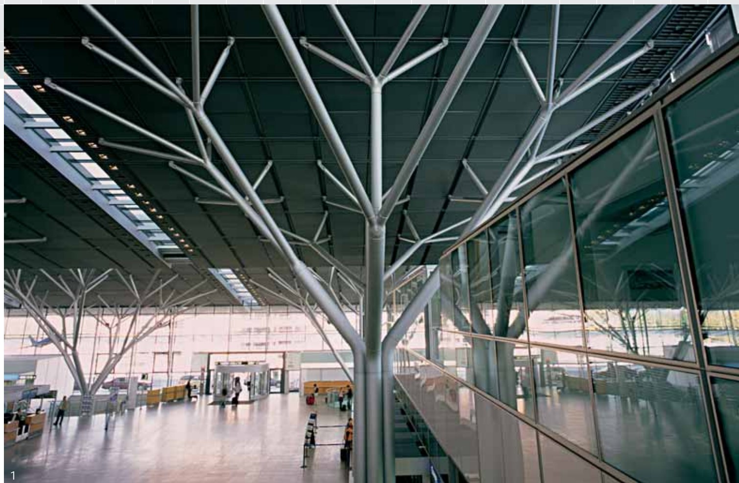
Ceilinglining 1 Aluminium full gratings Airport Stuttgart/Germany
