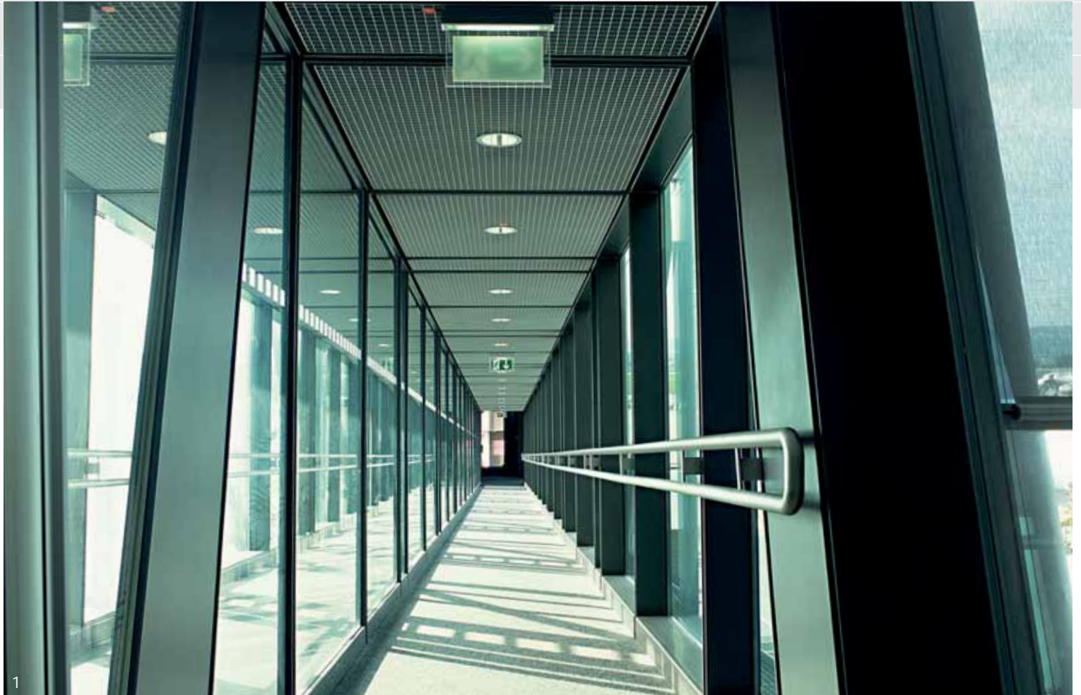
Suspended ceiling 1 Technical college Stuttgart/Germany
