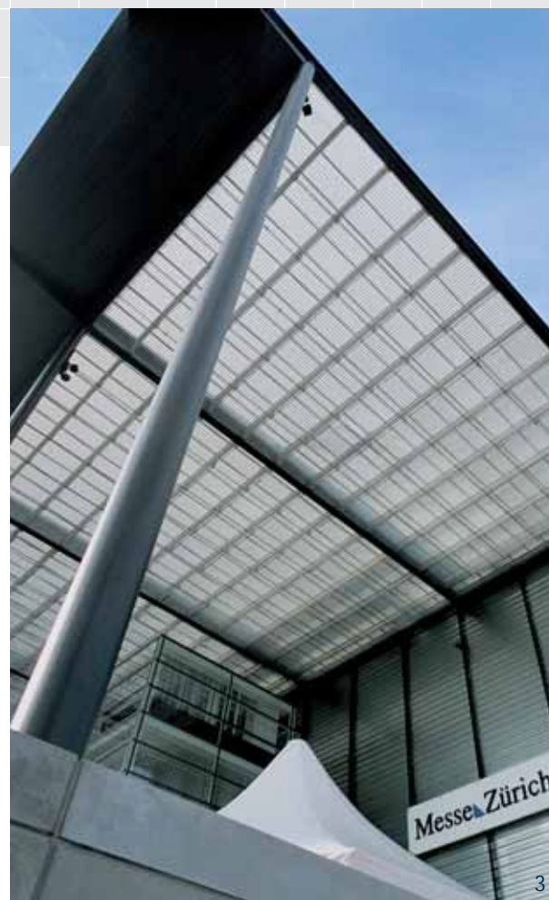
2 Suspended ceiling in stainless steel pickled press locked gratings Sony Center Berlin/Germany
